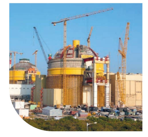
Construction site at Kudankulam nuclear power plant
