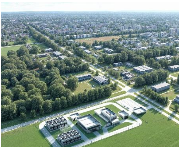
OTRERA plant located near suburban areas.
