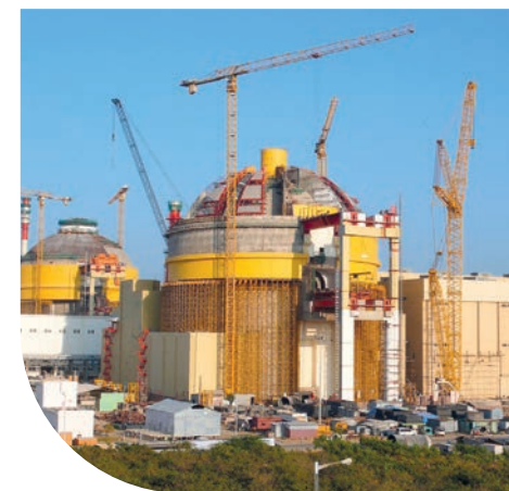
Construction site at Kudankulam nuclear power plant
